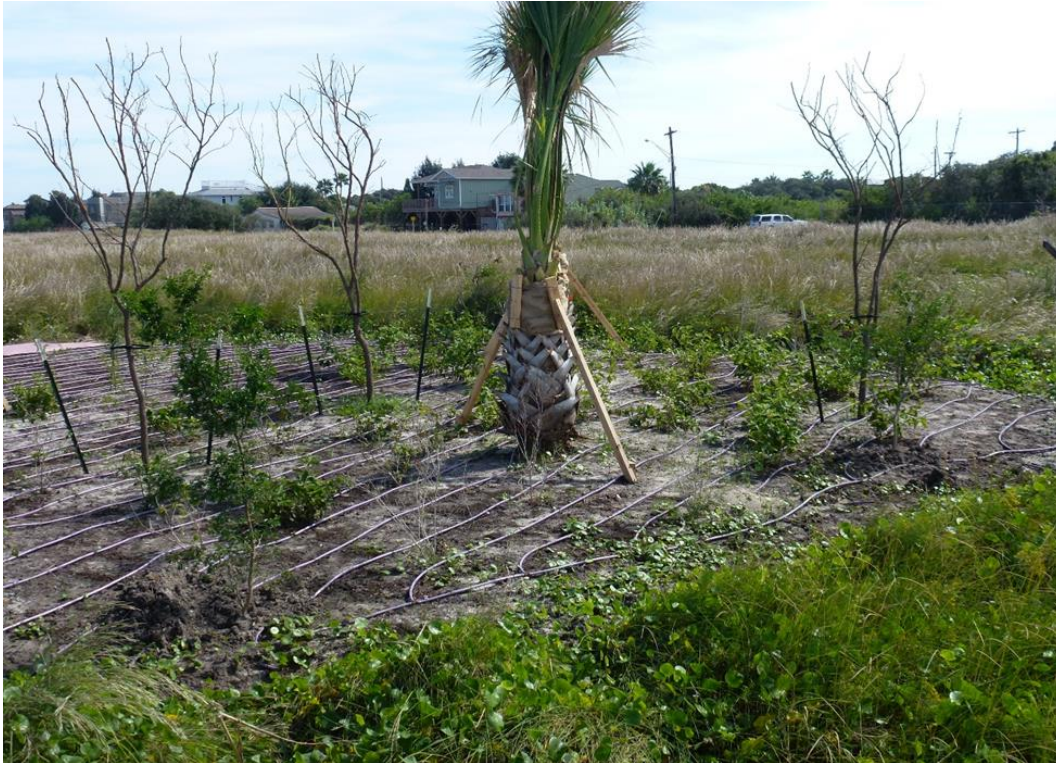
Photo 7. Drip irrigation lines installed on top of the weed barrier.
