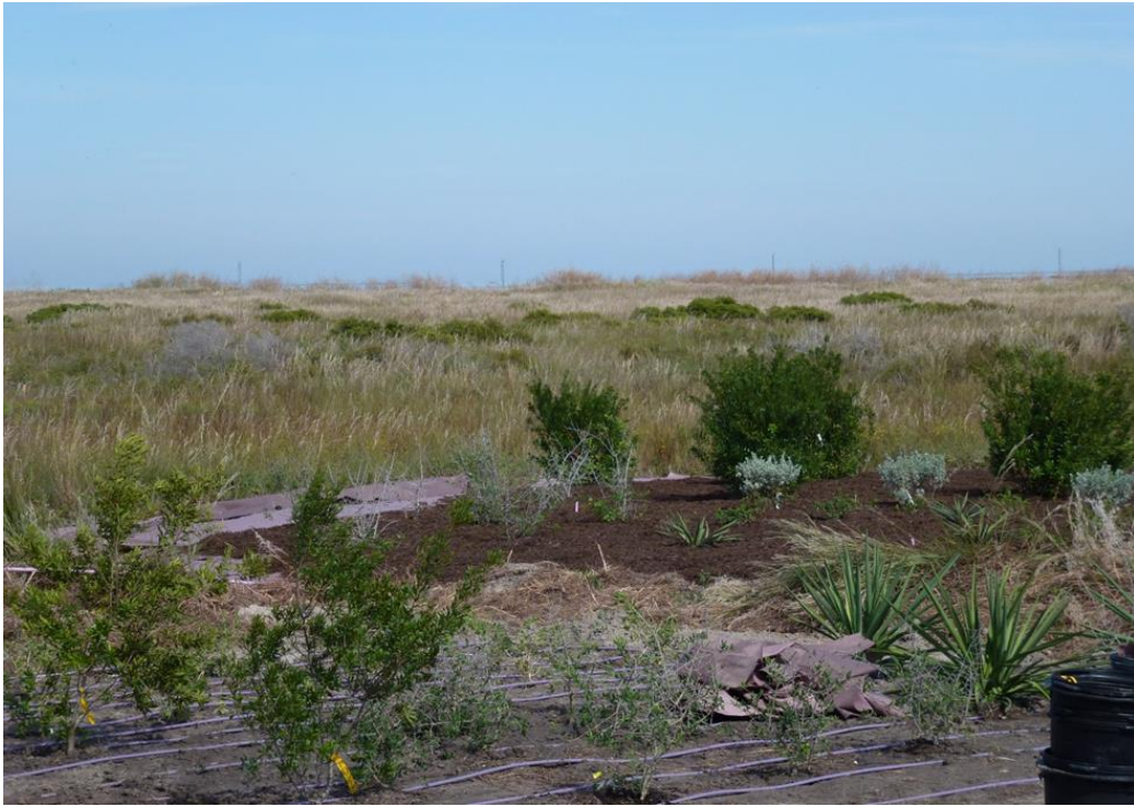
Photo 3. Construction included weed mats, mulch, and drip irrigation lines.
