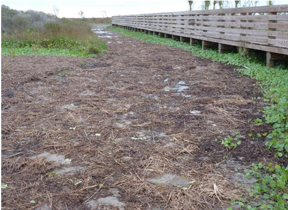
Photo 11. The stockpiled native vegetation/seed material was spread over the denuded areas.
