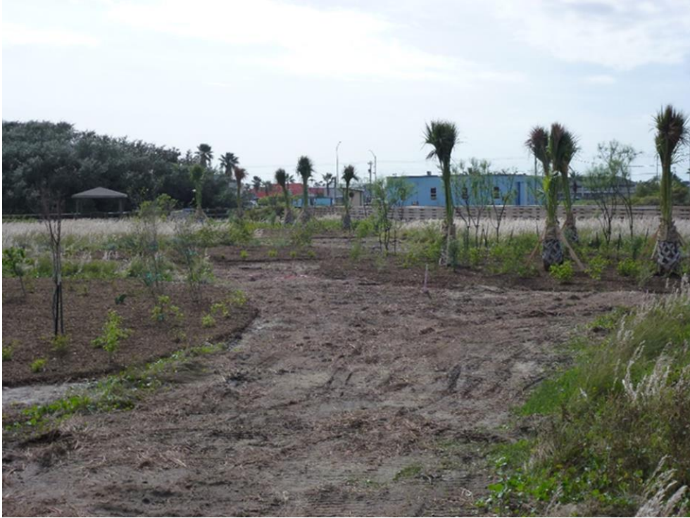
Photo 10. The site was restored by re-contouring rutted areas.
