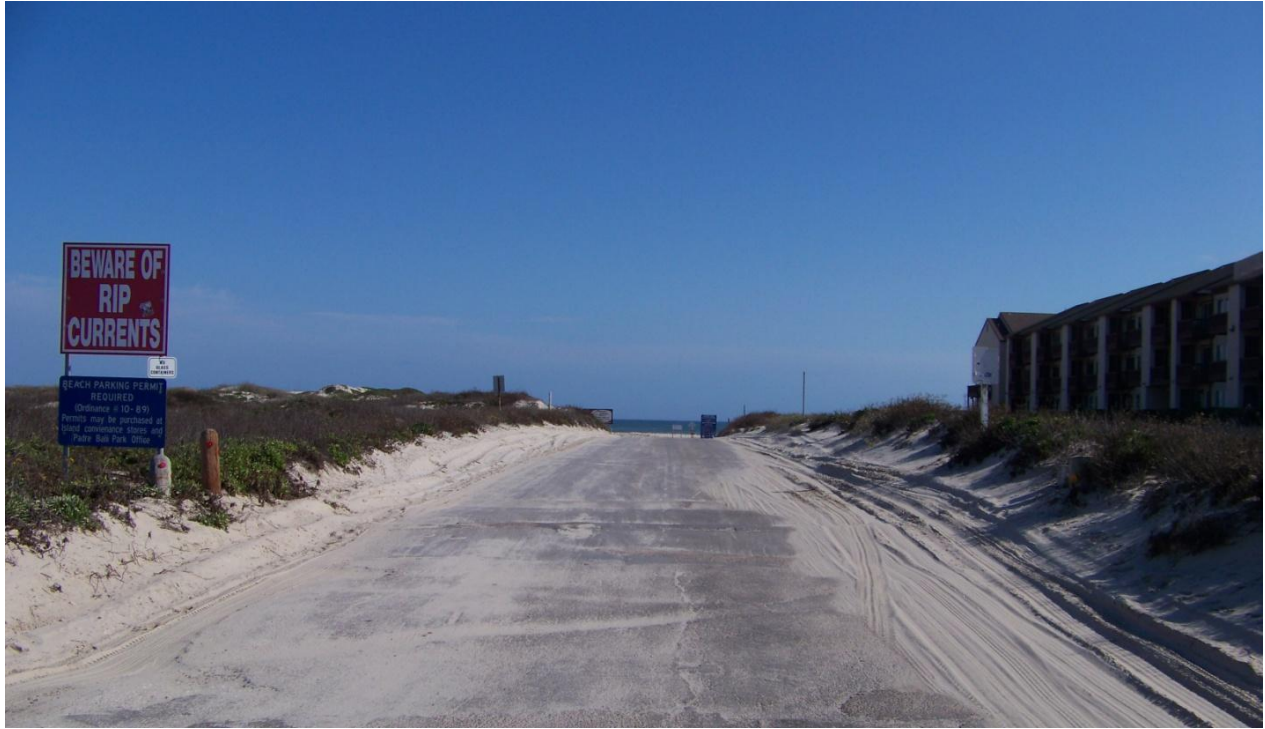
Figure 21: Beach Access Road 3A, Seaward View
