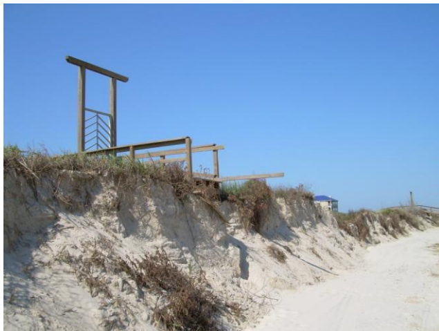
Figure 8: Hurricane Ike Dune Erosion
