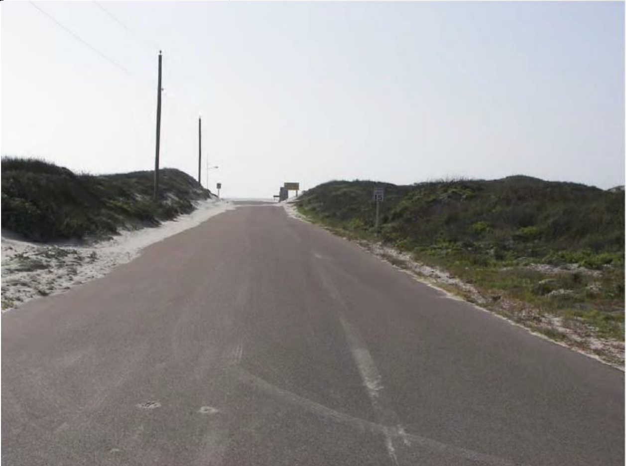
Figure 27: Beach Access Road 5, Seaward View
